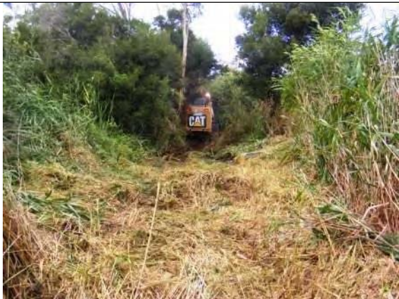
Commencing the connection to Swing Bridge Drive
